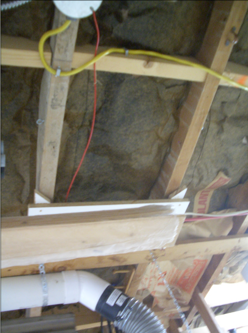
Figure 5 A rather blurry overhead shot of the lathe end of the pipe and its drop. Note the red wire: it is connected to a nut and bolt inside the pipe, and the bolt is secured to the pipe with another nut on the outside of the pipe, where the bolt exits the top of the pipe the red grounding wire is connected to the external nut using another nut. The wire is then attached to the metal junction box's ground wire. This is repeated at the other end of the pipe. Care was taken to ensure the wires inside the pipe never drooped into the pipe but rather ran tightly from bolt to bolt. This should minimize slow accumulation of particles and eventual blockages. Also, the internal wires were stripped of all insulation to increase static conduction.
